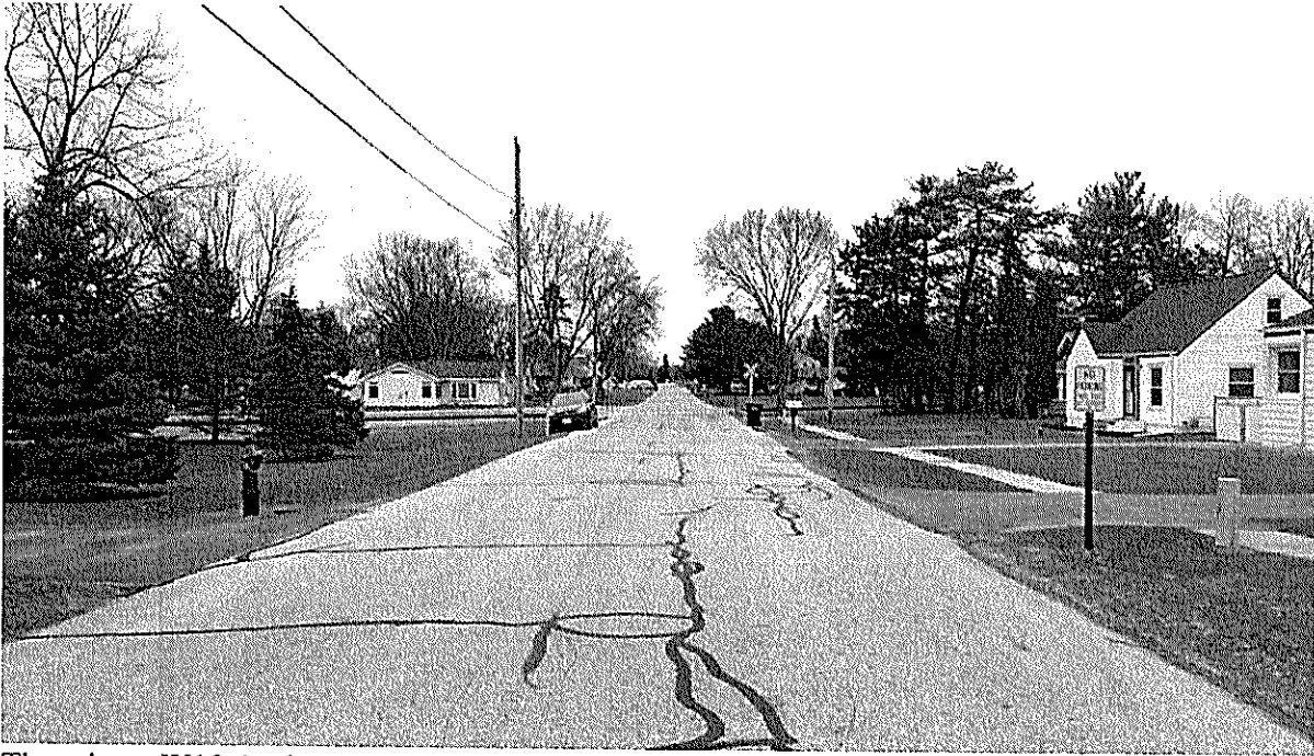
There is no W10-1 advance warning sign present on the southern approach.
