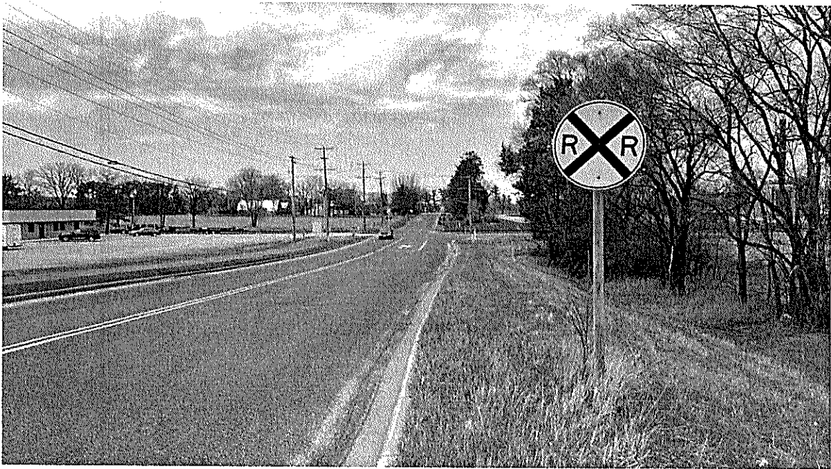
The northbound advance warning sign was located too far from the crossing.
