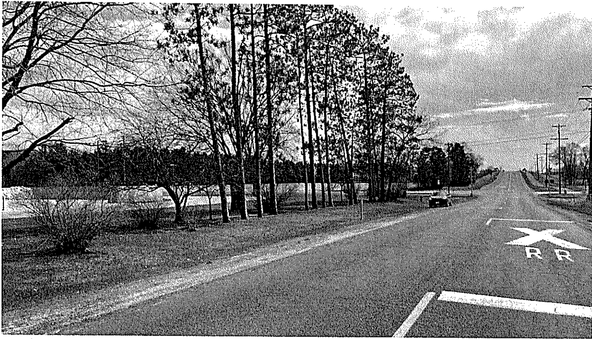
Brush on private property in the northeast quadrant is restricting highway users' view of the tracks from the southbound traffic lane.
