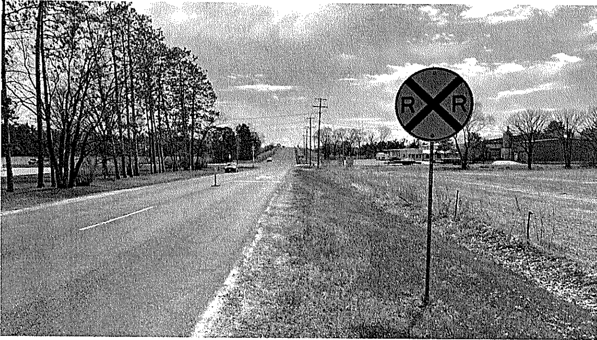
The southbound advance warning sign was located too far from the crossing.
