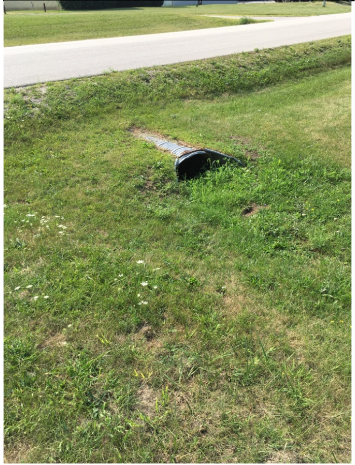
004 outlet clean needs excavation of s.ilt
