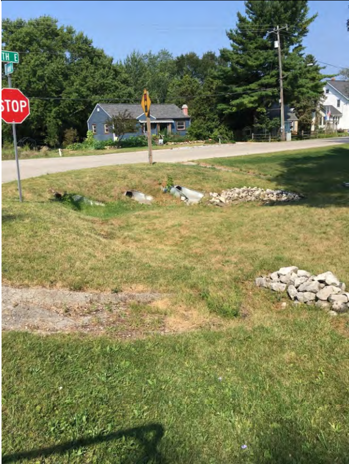
Looking east 3 red culvert. Needs clean out
