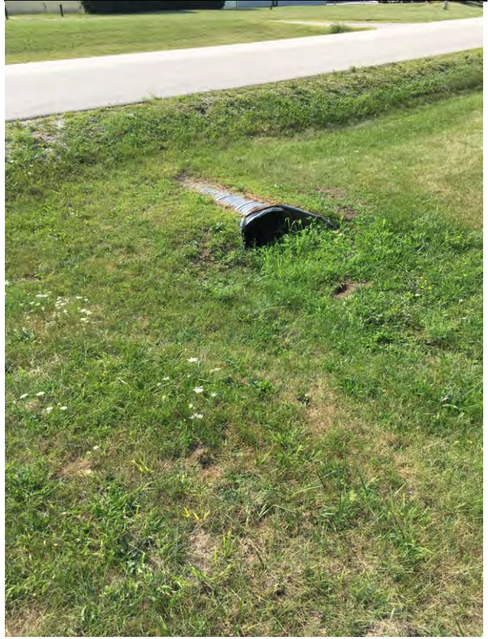
004 outlet clean needs excavation of s.ilt
