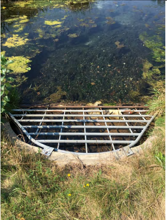
007 outfall looking west 18" depth @ pipe
