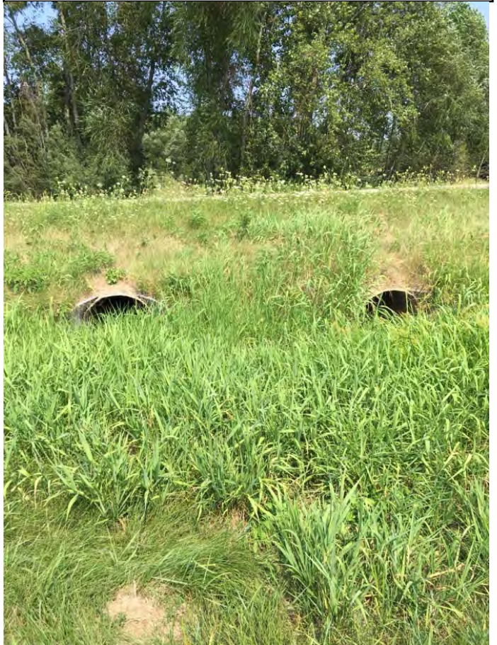
Outlet pipes south side need grass cleaned out
